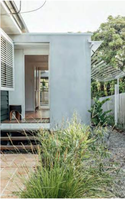
↑ A small addition to the western side of the house extends the living space and accommodates a laundry. Louvred 'vent boxes' to existing windows and adjustable slatted awnings provide shade.
